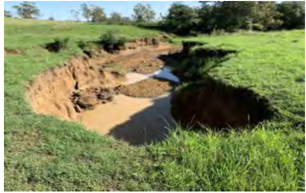
Channel joins dam at large eroded feature
